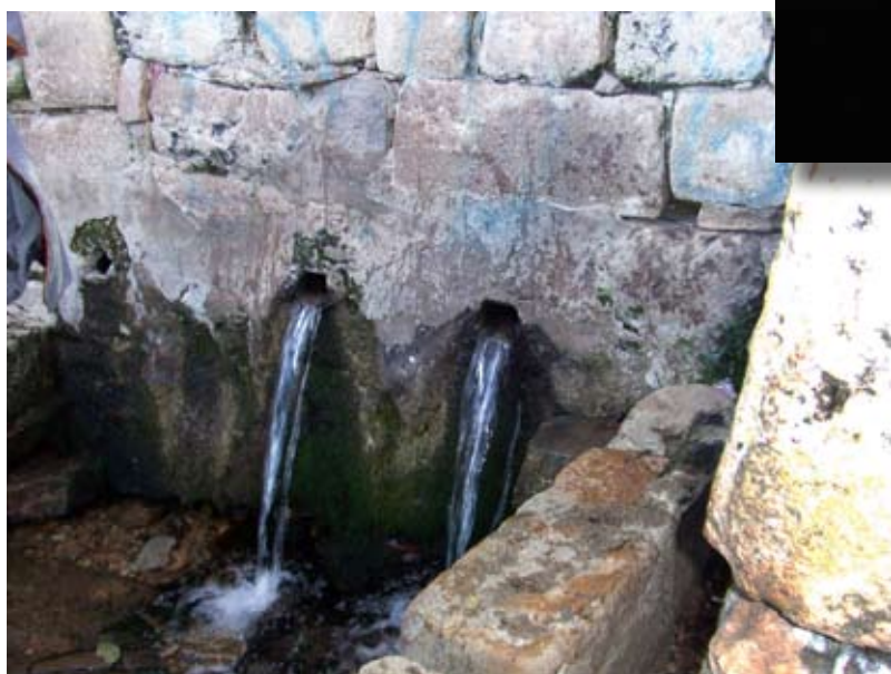
Water dumps rock
