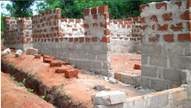
The new 2-block classrooms at Wonderful Love
